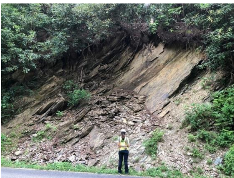
Figure 0.14. GRSM_051 located on Little River Gorge Rd is an ongoing wedge failure that is cleaned up annually. The red box indicates where this slope is in relation to the rest of the USMP inventory. Rock debris is continuously cleaned up and deposited on the opposite side of the road. Bottom Left photo credit: Thomas O’Shea, ETSU.
