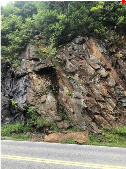
Figure 0.15. GRSM_013 on Newfound Gap Rd, located near Morton Overlook, a popular tourist spot. A 1.2m (4ft) rock can be seen in the ditch, that almost hit the road. Had this rock hit the road, traffic would have had to be diverted or closed as this is the only way up and down the mountain until Clingmans Dome. The red box indicates where the GRSM_013 is located. Bottom Left photo credit: Thomas O’Shea, ETSU.
