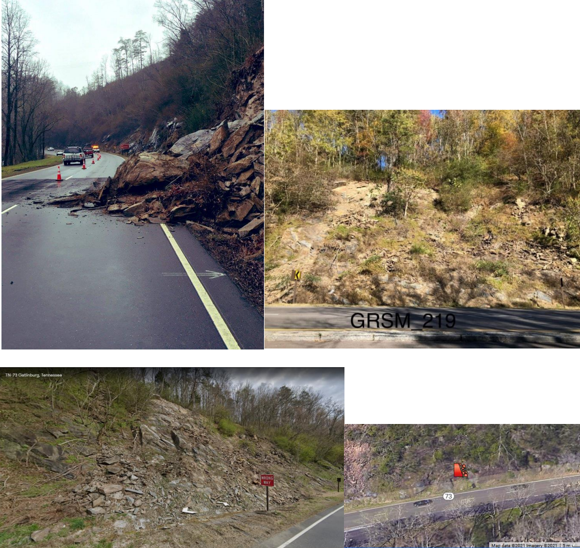
Figure 0.1. Top right: GRSM_219: the slope suspected to be the one that failed on February 12, 2021 on the Gatlinburg Spur. This slope received a poor rating (554) and was noted that previous wedge failures had occurred here. Bottom left: Google Earth image of GRSM_219 before failure. Bottom right: GRSM_219 shown on the interactive USMP database.
