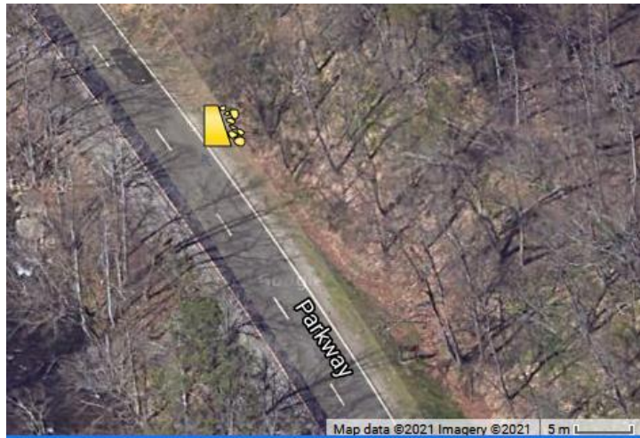
Figure 0.2. Left: Landslide that occurred on February 11, 2020 on Gatlinburg Spur in Great Smoky Mountains National Park. It was estimated by GRSM officials it would take 45 dump trucks to remove the estimated 500 cubic yards of material from the road. This slide did block both northbound lanes of the Spur. Photo: WJHL News (2020). Right: Samantha Farmer (researcher) in the process of rating GRSM_233, the mentioned above slope that failed. GRSM_233 received
