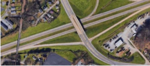
Fig. 4: Secondary location of the preliminary field-test (entrance ramp to US 321)
