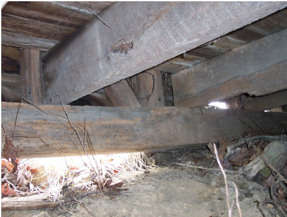
B6. Existing Construction & Condition of Floor System
