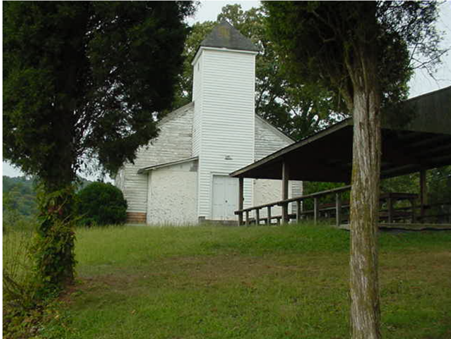
C1. Saunders Chapel (Front Façade)
