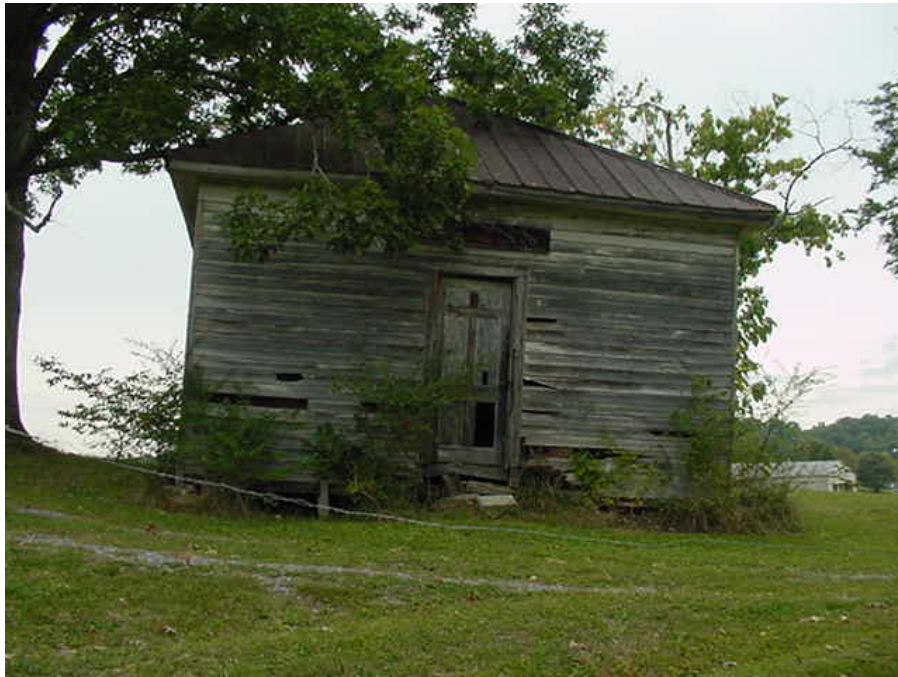
B1. Saunders Chapel School (Front Façade)
