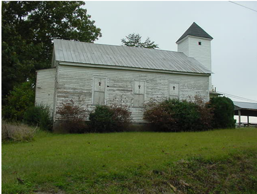
C3. Saunders Chapel (Side Façade)
