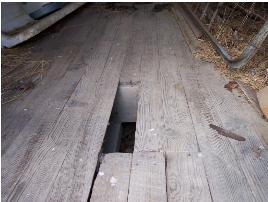
B8. Conditions at Interior, Floor System
