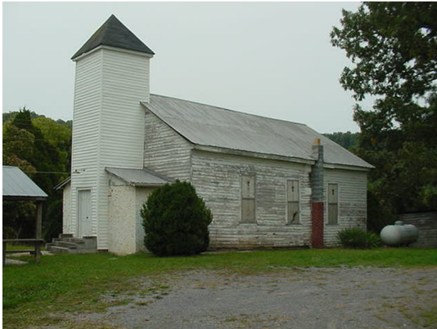
C2. Saunders Chapel (Side Façade)
