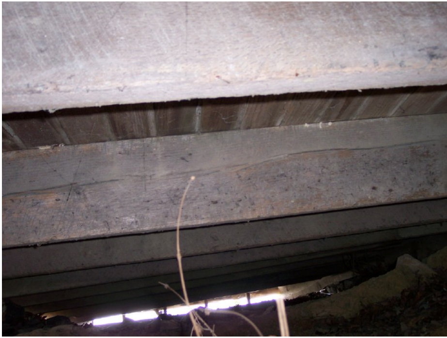
B7. Existing Construction & Condition of Floor System
