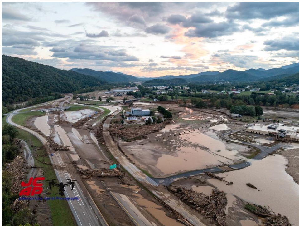
Area around the I-26 Jackson-Love Exit in Erwin, TN after the flood including the Unicoi County Hospital on the right side of the image. Source: Johnson City Aerial Photography
