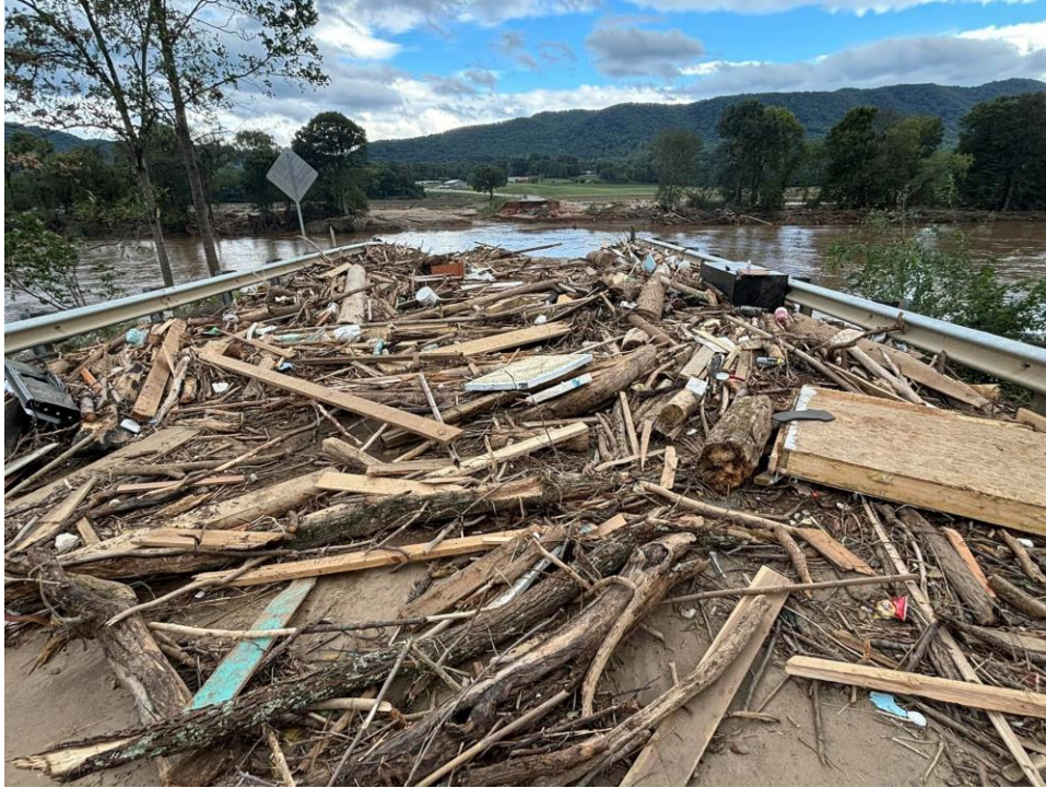
Debris near what was Taylors Bridge on State Route 81 in Washington County, TN Source: Facebook
