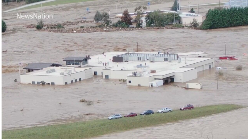
People waiting on the roof of Unicoi County Hospital, after the Nolichucky River inundated the building. Source: NewsNation
