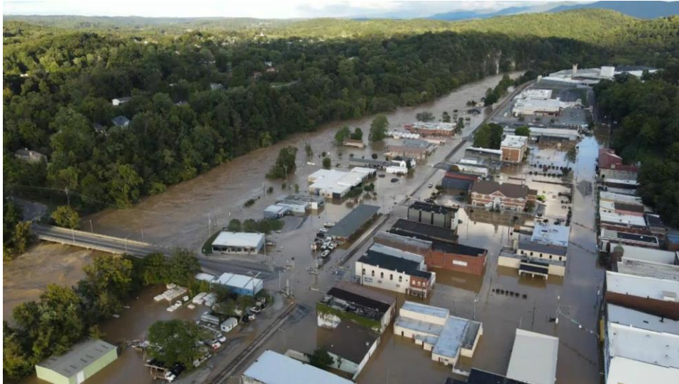
Downtown Newport, TN flooded by the Pigeon River. Source: WBIR
