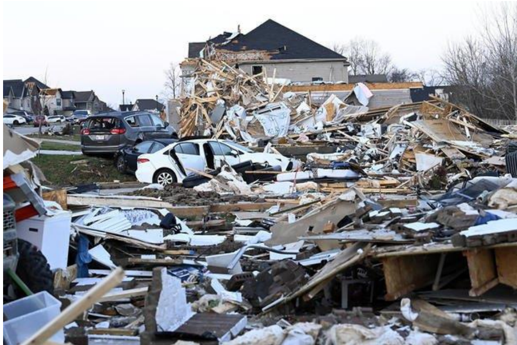
Damage caused by the tornado in Clarksville, TN. Image via: Mark Zaleski/AP Photo
