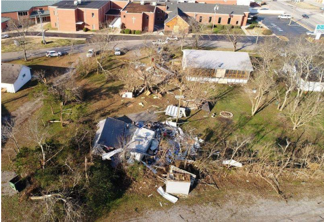
(Tornado damage in Gladeville (Rural Hill tornado); image from Wilson County Emergency Management Agency)
